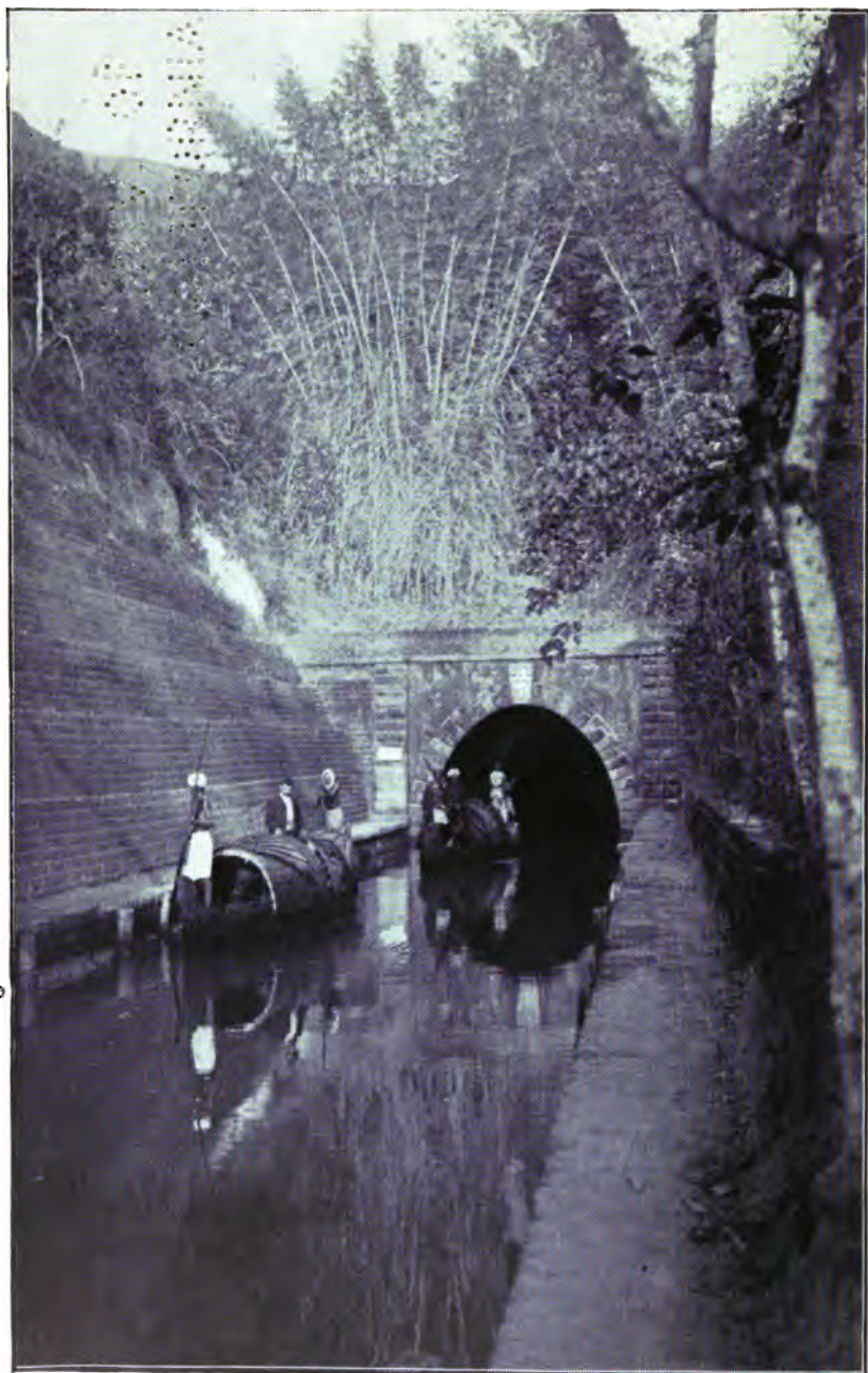
ENTRANCE TO A BOAT TUNNEL
